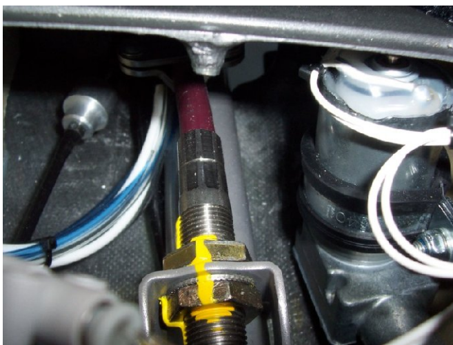
Fig 3 Pitch control cable in centre tunnel
